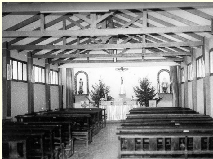
St. Elizabeth's Chapel in Rectory on Pidgeon Hill Road
